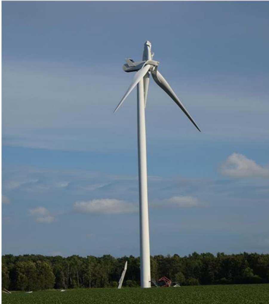
Skyway 8 wind turbine showing blade remnants, partial PowerCone device, and debris. [Photo: M.L. Morfitt]
